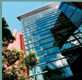
田 TE ARO CAMPUS ARCHITECTURE + DESIGN
